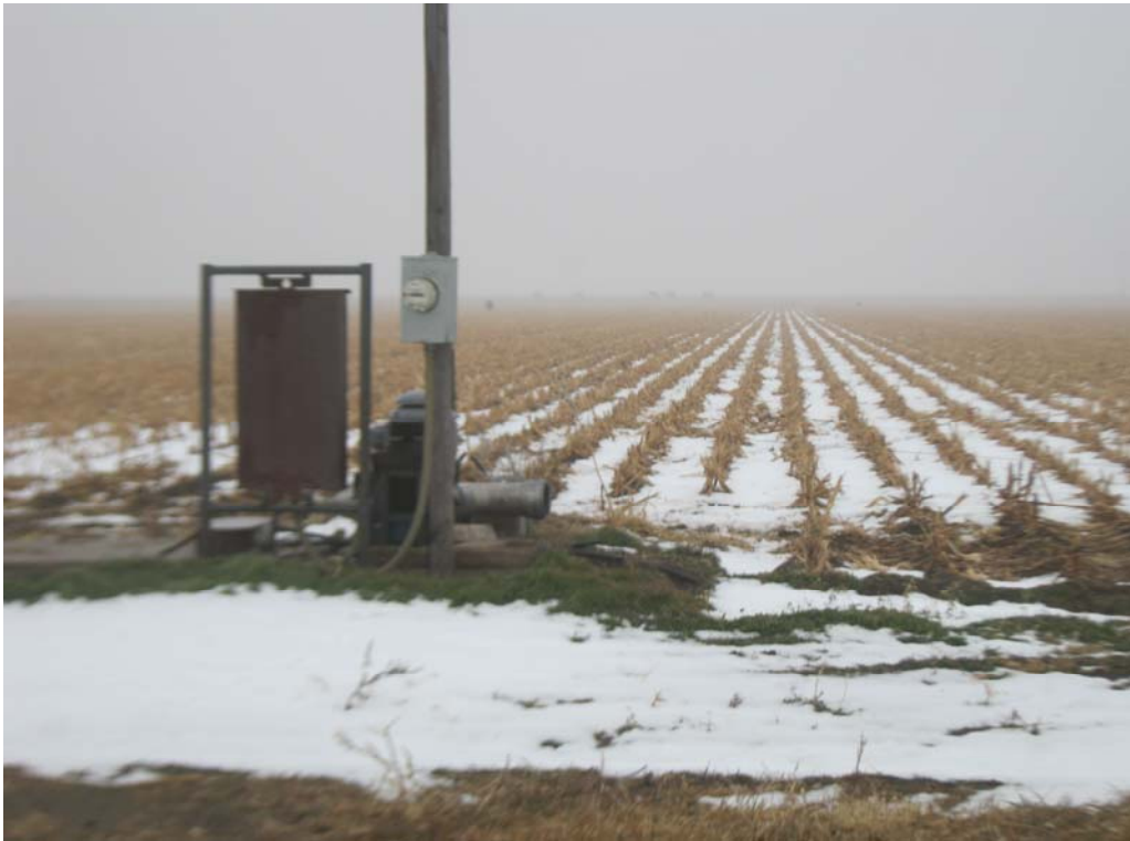
Photo 3: View of irrigation well located along 56 th Street.
