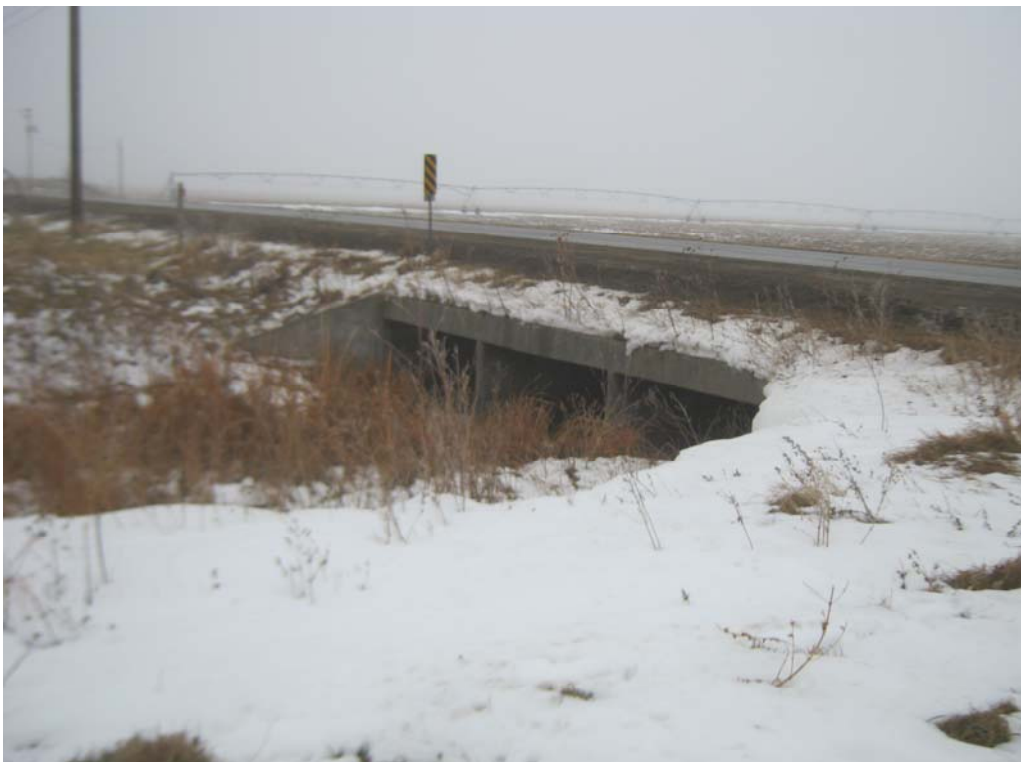
Photo 2: View of Antelope Avenue and drainage ditch, bordering the site to the south.
